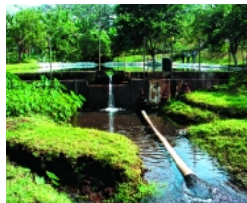
Decentral water purification plant.
